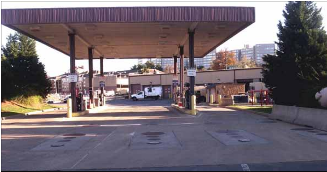
Arlington Fueling Infrastructure – Arlington made no changes to its existing fueling infrastructure except to thoroughly clean underground diesel storage tanks and add dispenser filters prior to receiving the first shipment of B20.
